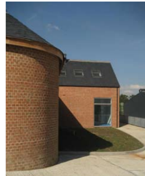
Right: The new farm buildings have been designed to enable the farm to be operated as an organic farm. Landscape around and between the buildings helps screen them and provide an attractive working environment.
