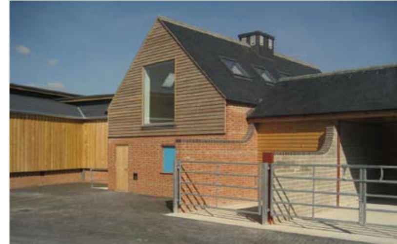
Above and below: Existing farm buildings rebuilt, and refurbished to provide the farm office, staff welfare, stores and visitor facilities together with small animal pens Full height window on the first floor admits daylight to the interior space on both elevations
