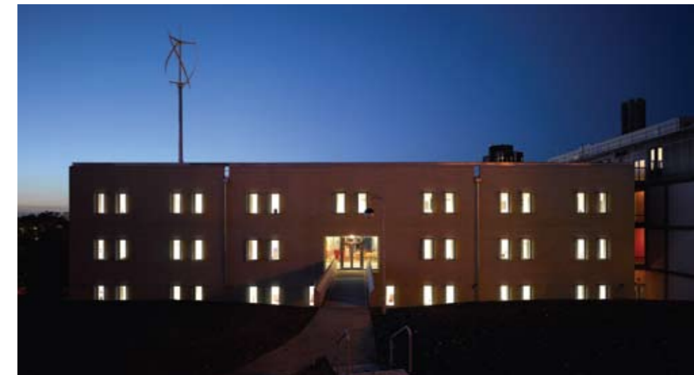
Right: A simply articulated composition playing off the 'private' paired study windows with the bay wide 'public' entrance
