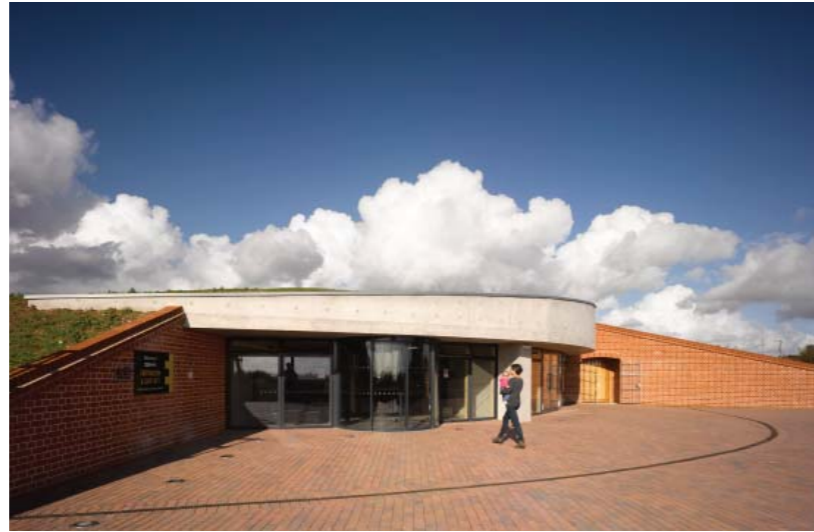
Right: The entrance to the new visitor centre. Below (top): The cafe and shop in the new visitor centres. Below (bottom): The new earth covered visitors centre.
