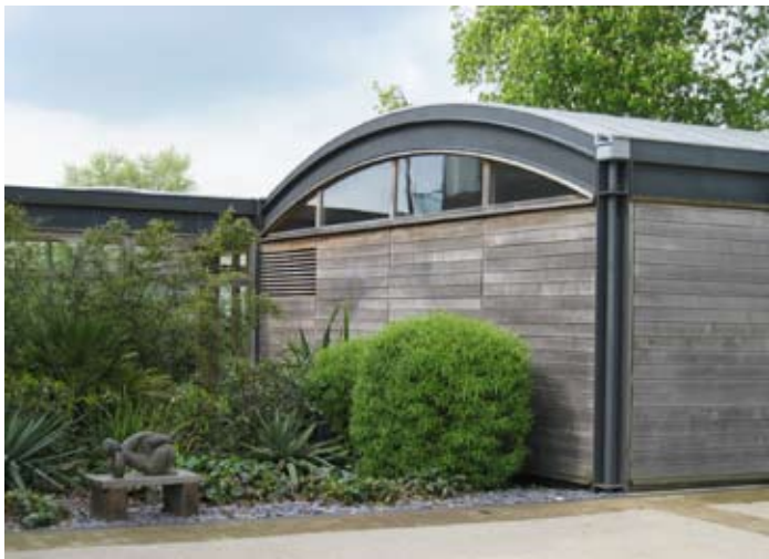
Above, top: section showing canopy and central circulation system Above: landscaped courtyard
